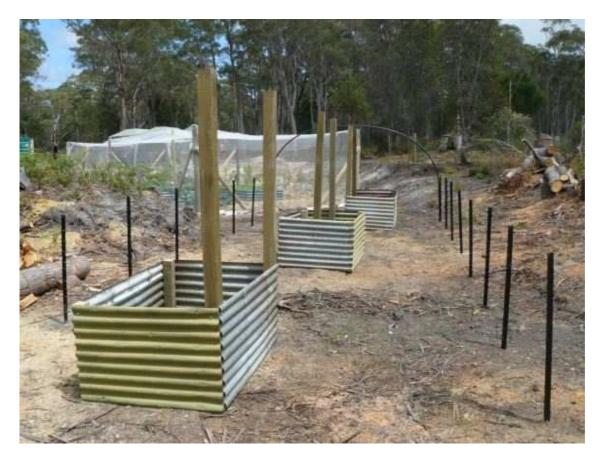
Once the pickets were in place we made three raised beds from recycled roofing iron to hold the posts in position. This was easier and more eco friendly than concreting them in place. The beds not only hold the posts but provide weight to stabilise the frame in strong winds.
