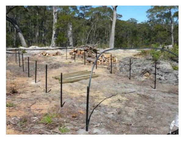
After laying out the position of the star pickets we couldn't bash them in and had to drill into solid rock with a masonry bit. This took all day, plus 20 Anzac biscuits and several cups of tea!!! There are eight arches altogether giving us 10.5m in length and 4m wide, 42sqm in total.
