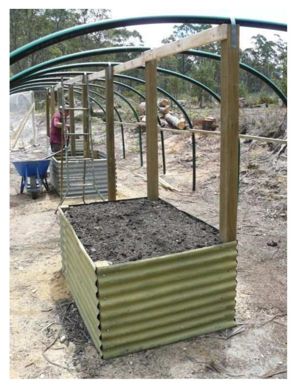
This shot shows the bracing. We have used 75x38mm pine for the side rails that was left over from another job, and 90x45mm merchant grade pine for the top rail. We decided to use some brace strapping to hold the pipes to the posts as this gives a seamless outline for the plastic and the top rails on their sides will provide ample places for hanging pots.
