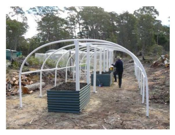
After we had finished the frame we painted it white using left over paint given to us by a friend (thanks Tim). We did this to reflect the sunlight from the black tubing and metal straps so it stays cooler and doesn't affect the plastic over time.
