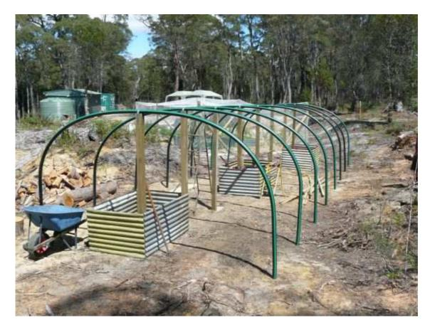
We cut the tubing into seven metre lengths and pushed it down onto the pickets, this is a two person job, but was fairly easy to do. Instant frame!! We were very impressed with the strength of the frame already, and we hadn't even put the timber bracing on. You could use this frame for many applications and Nev is planning structures all around the place much to Bryon's disgust.
