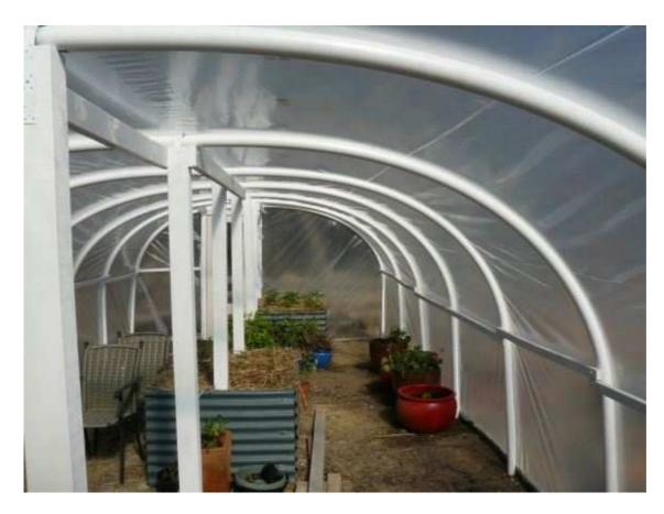
The next step was putting the plastic on. A 25m roll of poly-tunnel plastic cost \$208 from Waratah Distributors in Launceston. It is 7.5m wide to suit the 7m arches and is made from a UV stable non-rip plastic. It is important to get the right plastic as some tear very easily and also break down rapidly in the sun. Some I bought for a cold frame previously only lasted one season. The supplier indicated this stuff should last at least five years and it is very hard to tear.
